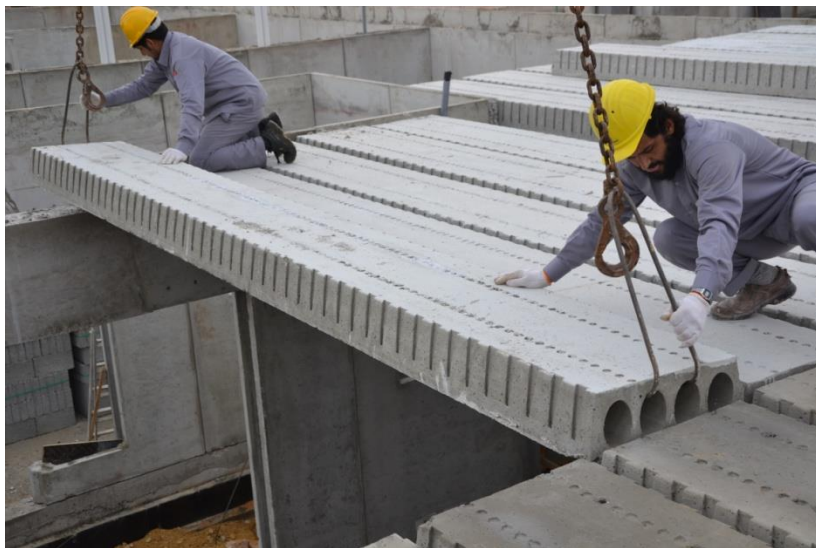
HCS with toothed shear key installation
