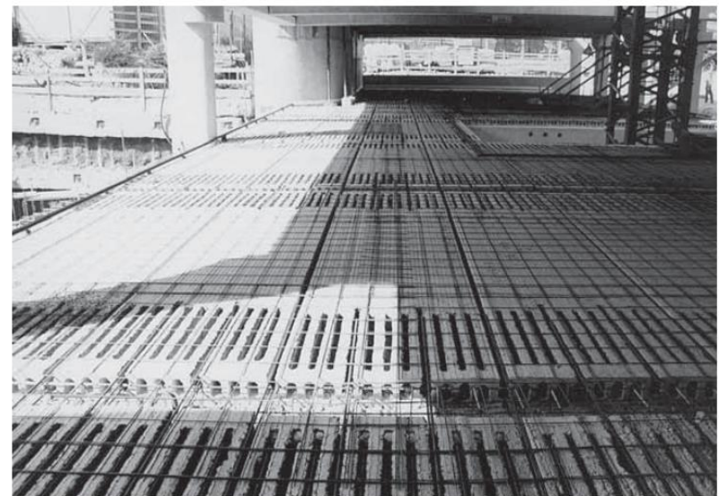
Diaphragm behaviour of HCS floor
